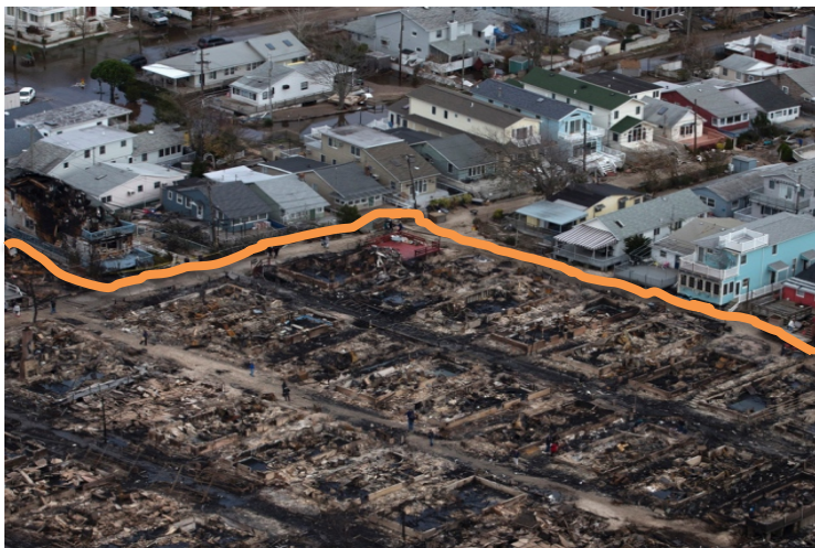
Aerial shot shows the burned remains of homes at a beachfront neighborhood in Queens. More than 100 homes in the community were completely destroyed by fires during super storm Sandy.
